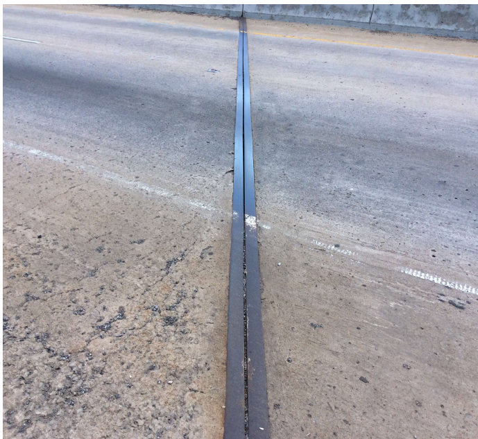
PHOTO 3 Description Expansion joint over Bent 3.
