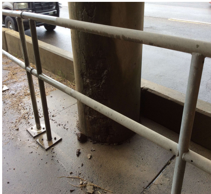
PHOTO 1 Description Bent #2 Column #1 Spalling with exposed reinforcing steel
