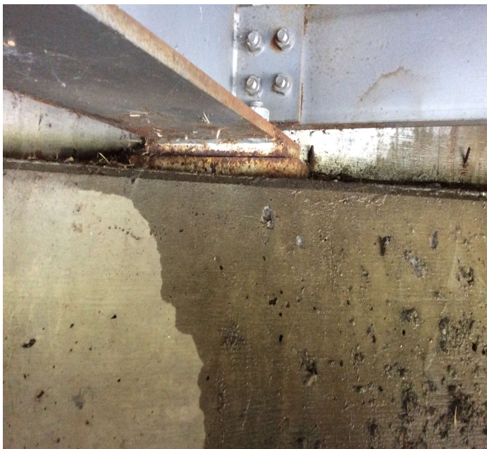
PHOTO 1 Description Bent # 1 Beam # 7 Active corrosion in the bearings
