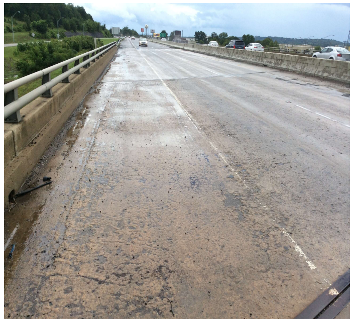
PHOTO 2 Description Span # 1 Scale in the driving surface
