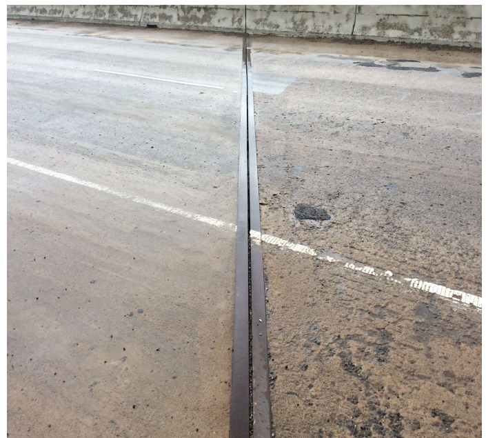
PHOTO 2 Description Bent # 2 Missing joint seal.
