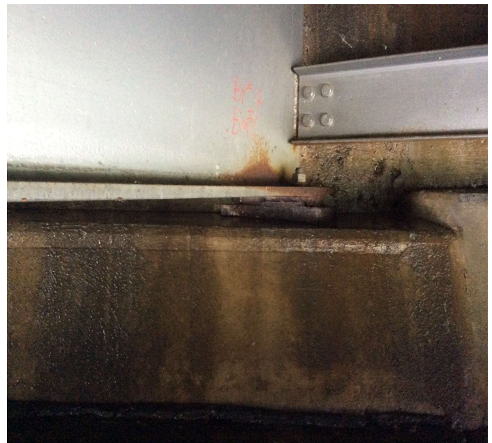
PHOTO 2 Description Bent # 4 Beam # 6 Active corrosion in the bearings.
