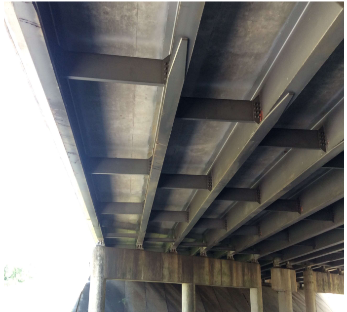
PHOTO 2 Description Span 2. Insignificant scrape marks due to traffic impacts.
