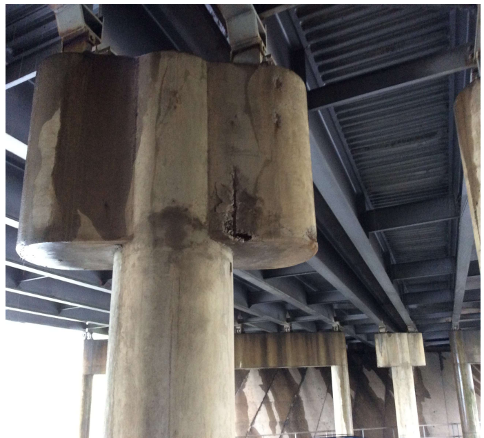
PHOTO 2 Description Bent #3 Column #4 Spalling with exposed reinforcing steel.
