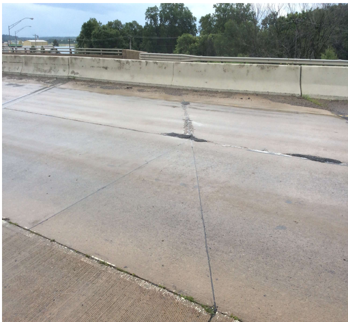
PHOTO 1 Description Bent # 1 Approach slab spalling
