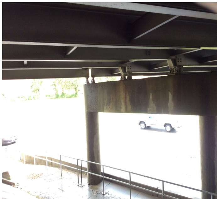
PHOTO 1 Description Bent # 2 Joint leakage
