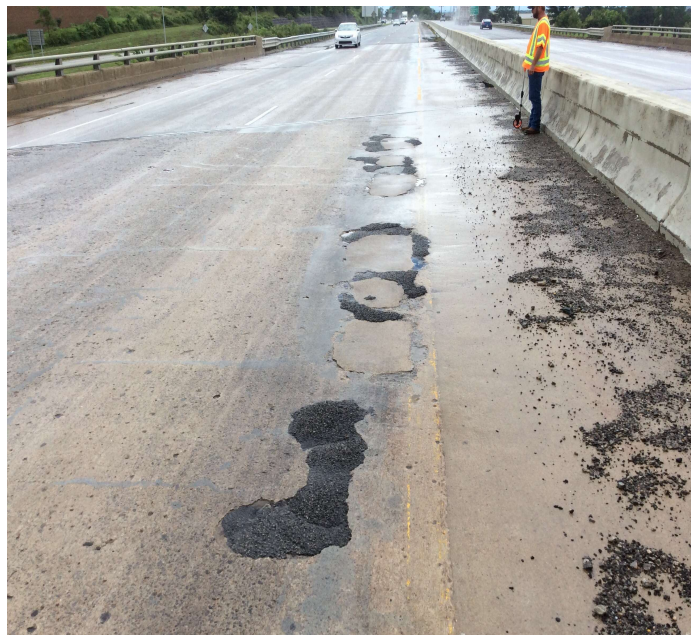
PHOTO 1 Description Span # 1 Pothole repairs
